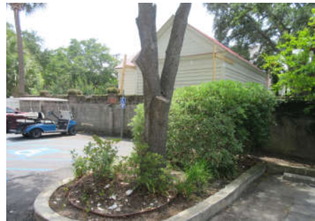
Irrigation sprinkler lines probably should be buried underground.
