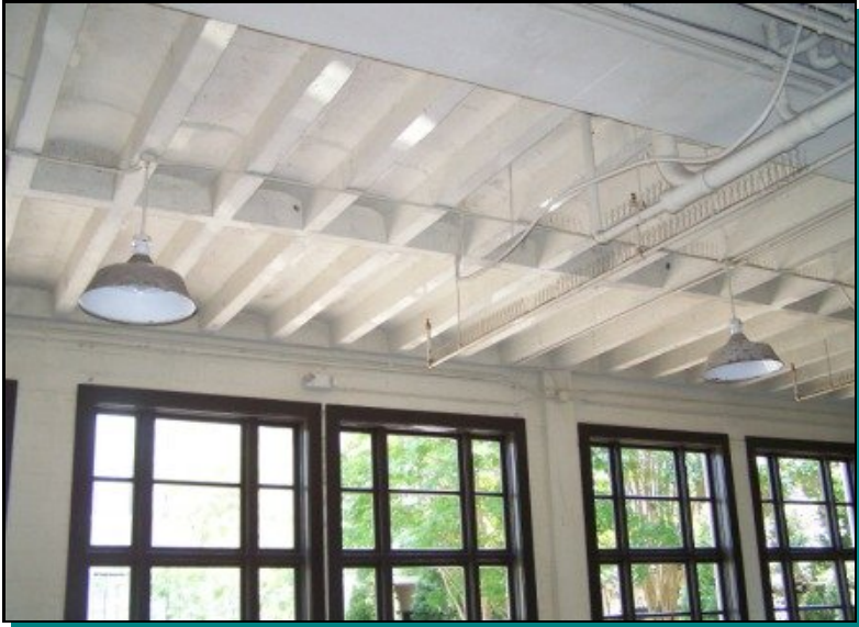
Garage light fixtures
