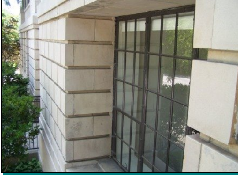
Paint finish on metal windows
