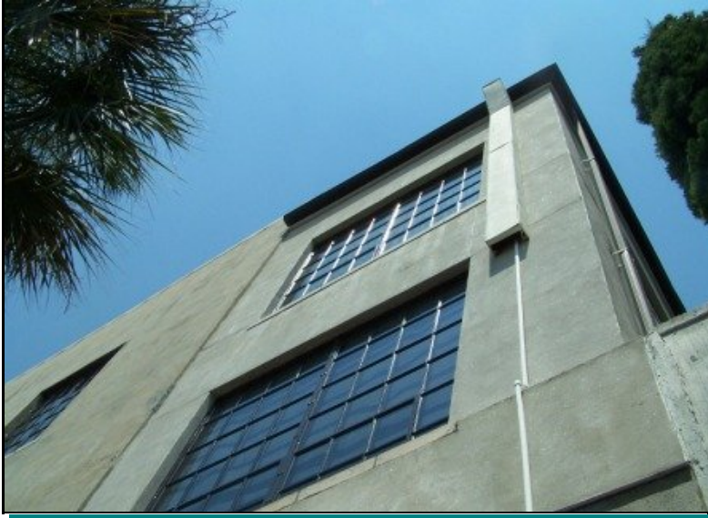
Gutters and downspouts
