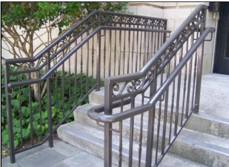
Paint finish on metal rails
