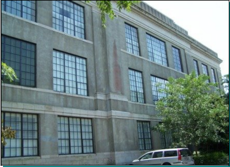
Side elevation, Main Building
