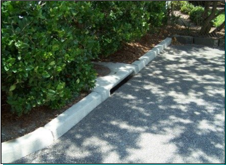
Catch basin and concrete curbs
