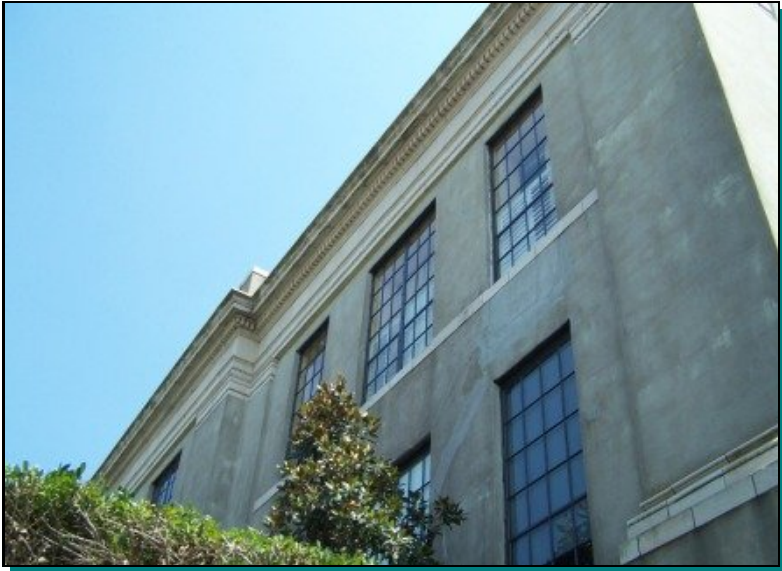
Rear elevation, Main Building
